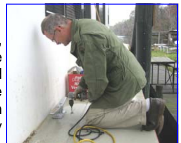
Steve drilling for the cleat
