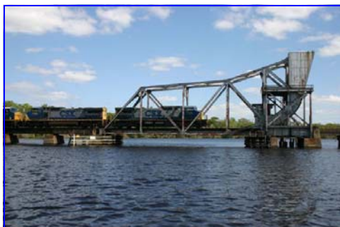
Train on Buffalo Bluff Bridge
