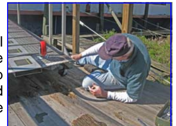
Joe Morris replacing casters
