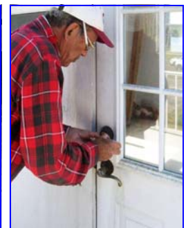
Bob Trail repairing latch
